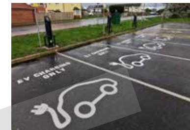
EV Chargers, Lynnsport
